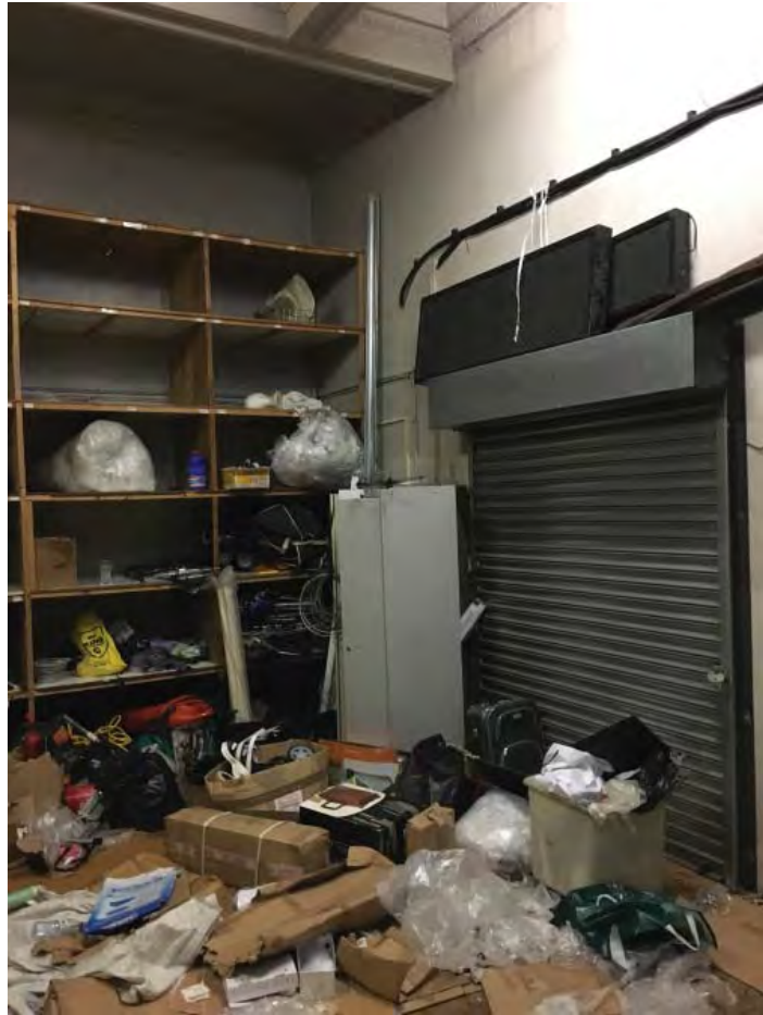
13. Rear storage area of no. 245 High Road. Existing roller shutter between units of 245 -247 & 249.
