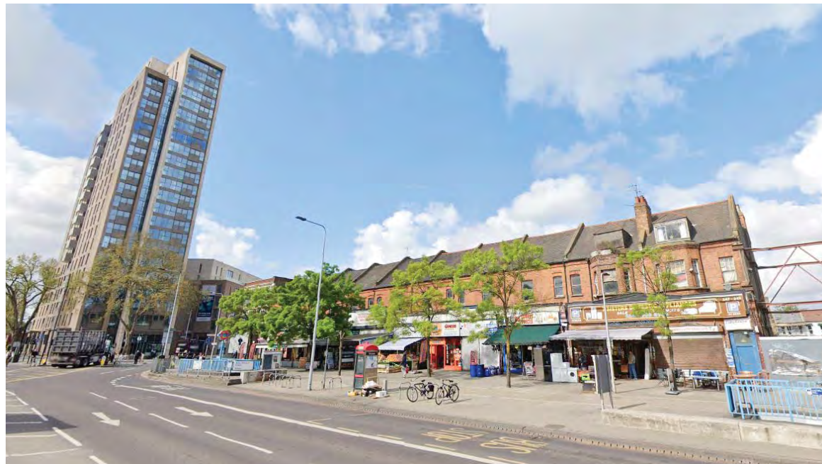
6. View of a portion of the wider terrace 227-249 High Road looking South-westwards towards the recently constructed 22 storey Apex House. The existing canted bays of 247 -249 are visible (right).
